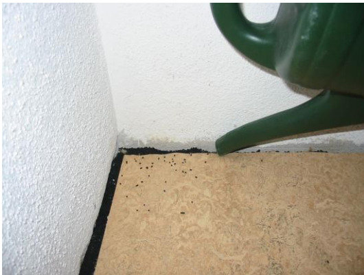
Abb. 2: Körniges Adsorbens = Gasfilter
